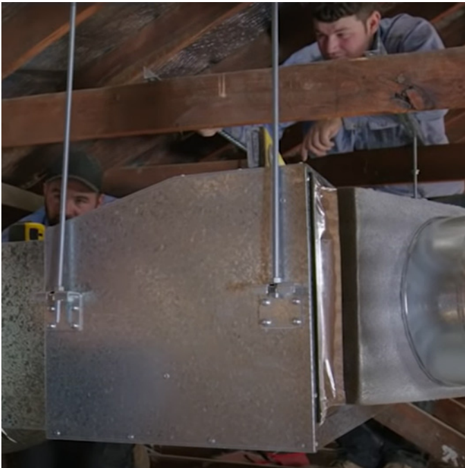
Installation with threaded rod (traditional method)
